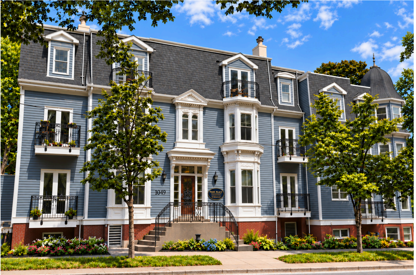
South Park Street view
